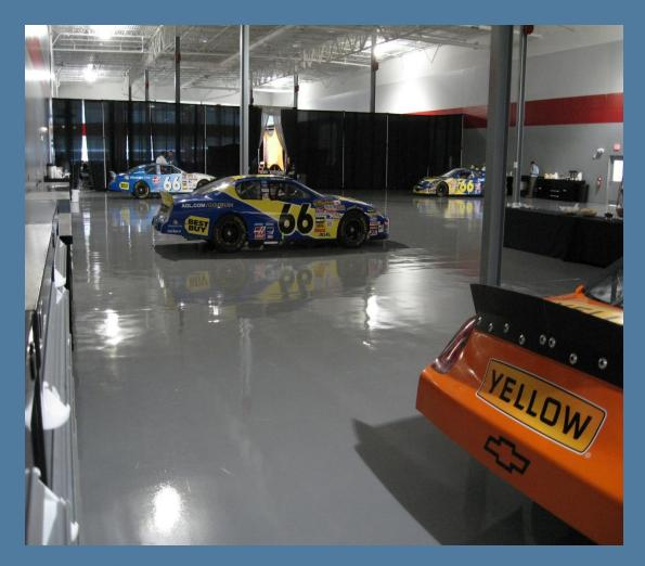
Stonclad GR, an epoxy mortar that uses 30% recycled glass filler and a rapidly renewable soy-based component
